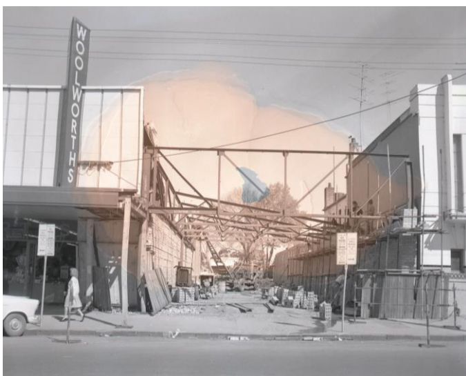
Removal of Central Stores & new build – October 1965. Note: 1. Bluestone curbing still in Murray Street. 2. Eastern wall of the Union Club Hotel to the right. Image - CDHS - Bela Bard Brucker collection
